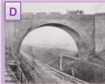
**D** The lofty and well-built arches support the tracks of the Midland Railway. Originally a two-track railway, the join to the later-constructed additional tracks can be clearly seen. Photo shows the earliest structure with branch line beneath. *COURTESY ST ALBANS' MUSEUMS.*
