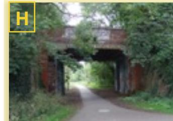
The original narrow arched road bridge of Cottonmill Lane was replaced shortly before the end of passenger services. Notice the change of brickwork on the abutments, to accommodate a wider roadway.
